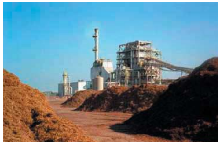
Figure 5 – Commercial biomass power plant
